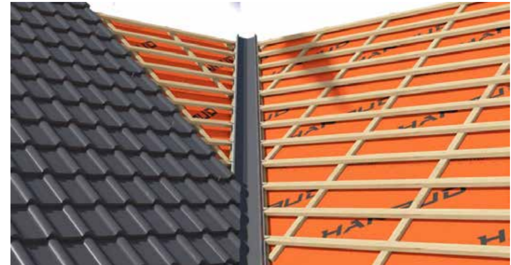
Fig. 17 Laying of roofing sheets at the basket gutter.
