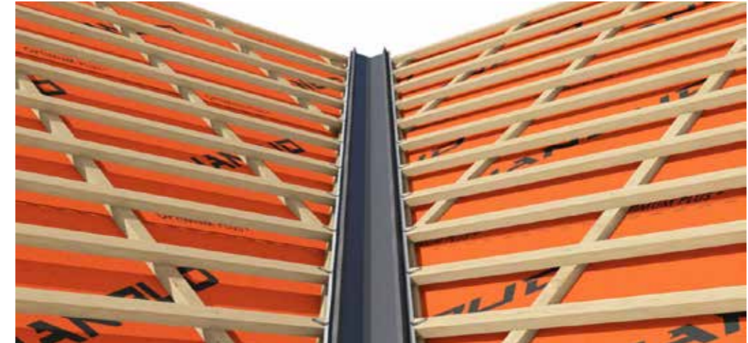
Fig. 12 Installation of basket gutter.
