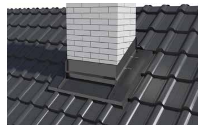
Fig. 22 Fixing the top flashings to the chimney with dowels.
