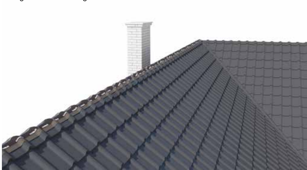
Fig. 23 Installation of ridge tape.
