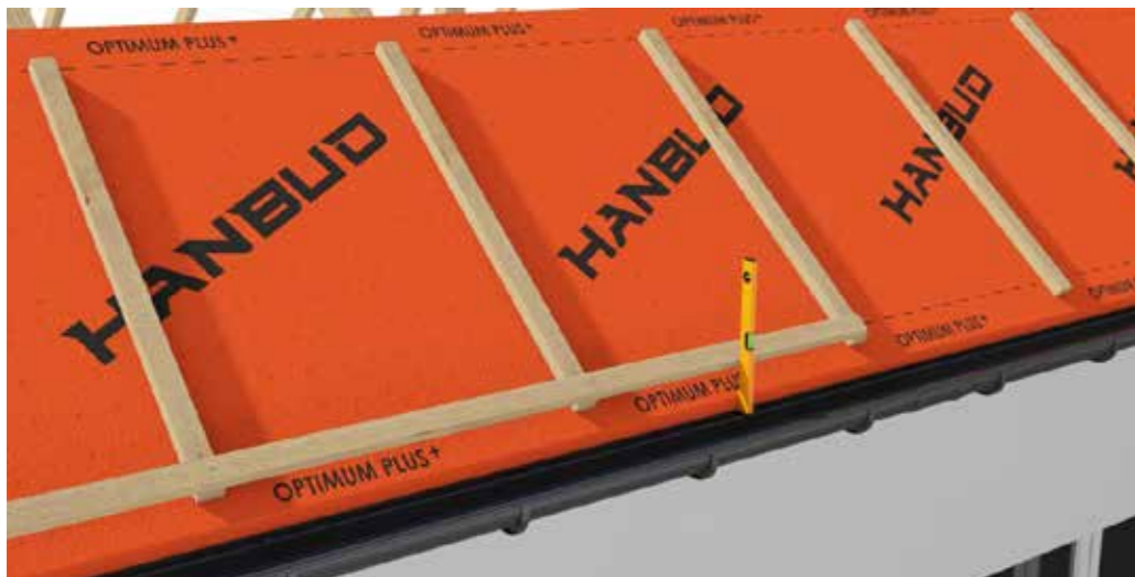
Fig. 7 Installation of counter-battens on the roof slope.
